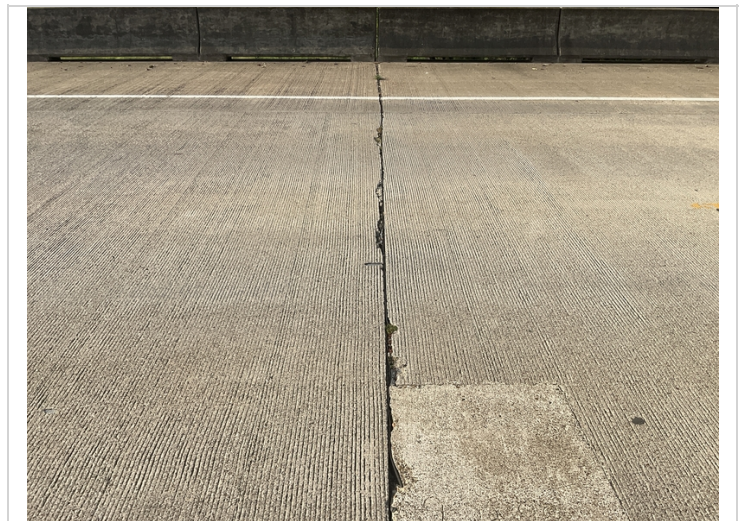
07/22 joints need cleaned and resealed
