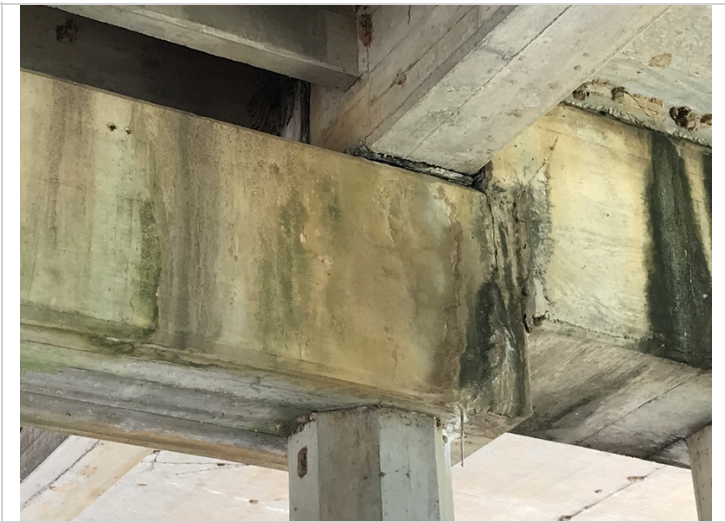
Bent 4 cracks in RCDG and cap
