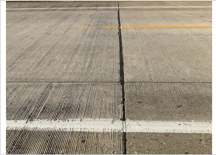
07/22 joints need cleaned and resealed
