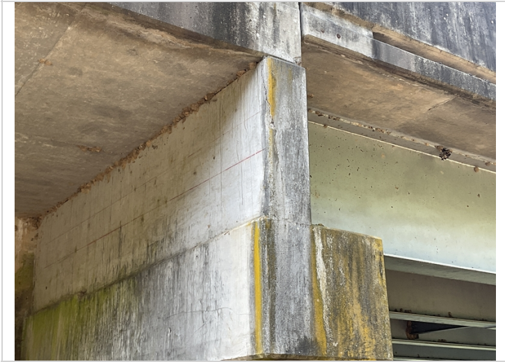
07/22 bent 8 cracking left side top of cap
