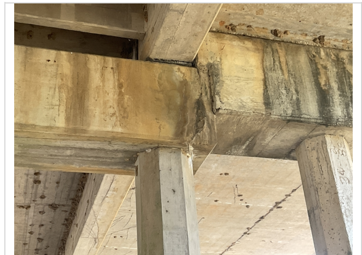
07/22 cracking with efflorescence on bent 4 center cap top right corner
