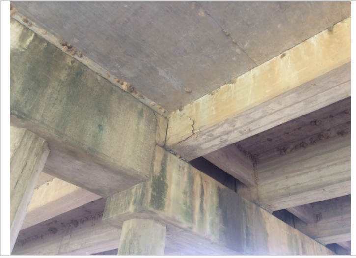
SPAN 7 CRACK IN GIRDER
