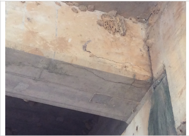
CRACKING BOTTOM OF GIRDER SPAN 9
