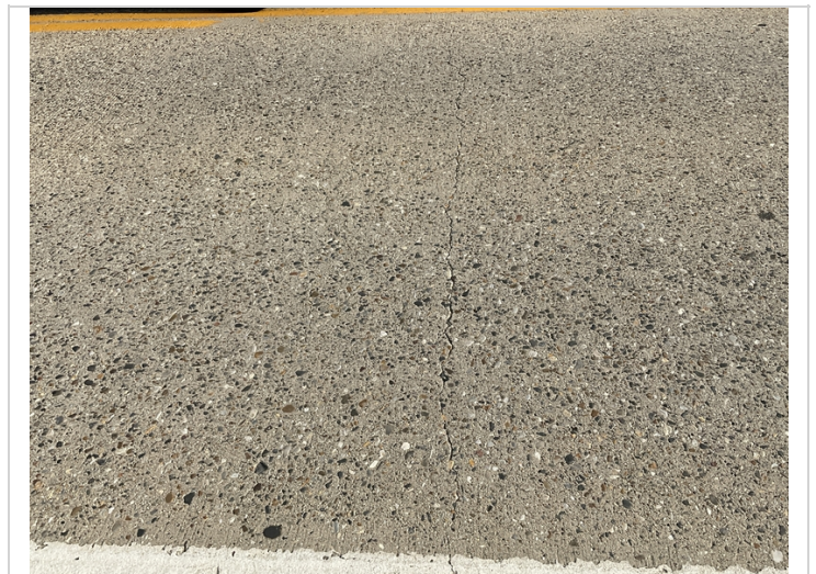
07/22 cracking in deck
