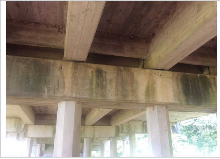
CRACKING TOP OF CAP BENT 8
