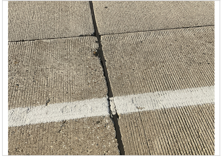
07/22 cracking in deck
