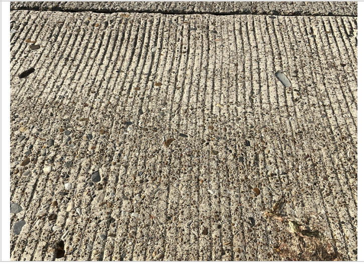
07/22 hairline map like cracking in deck
