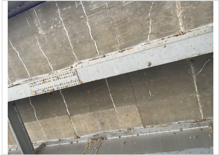
Efflorescence on underside of deck at various locations all spans
