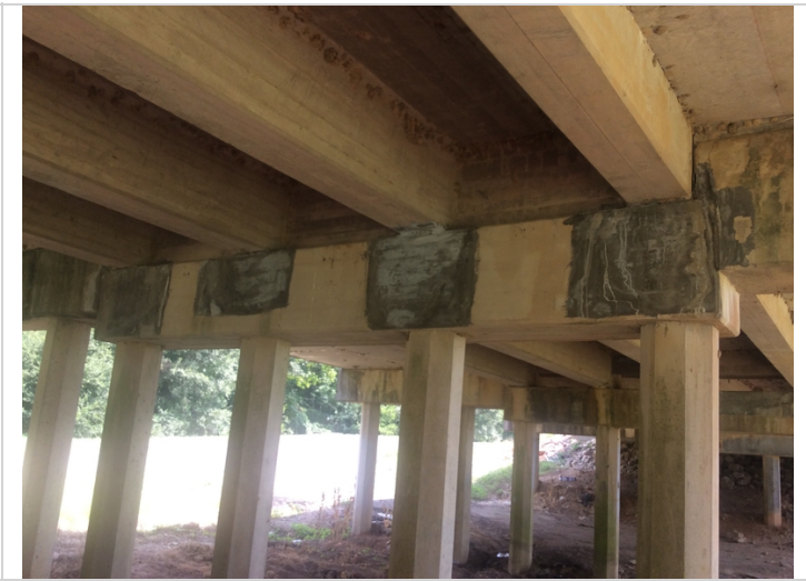
REPAIR WORK DONE BENT 9
