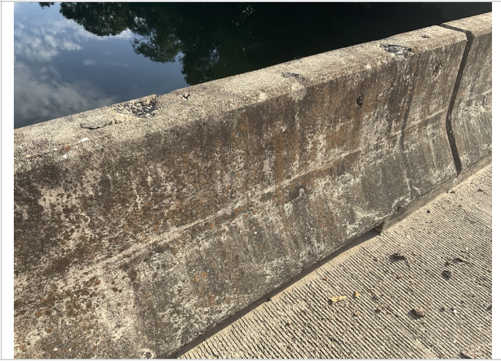
07/22 spalls in parapet wall
