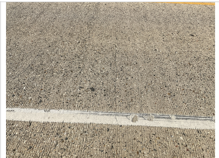
07/22 cracking in deck
