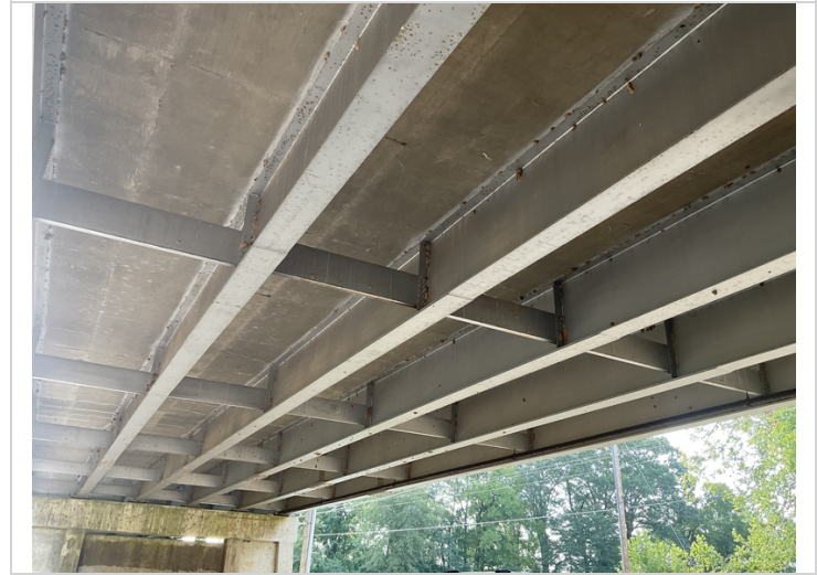
07/22 Typical superstructure of main deck
