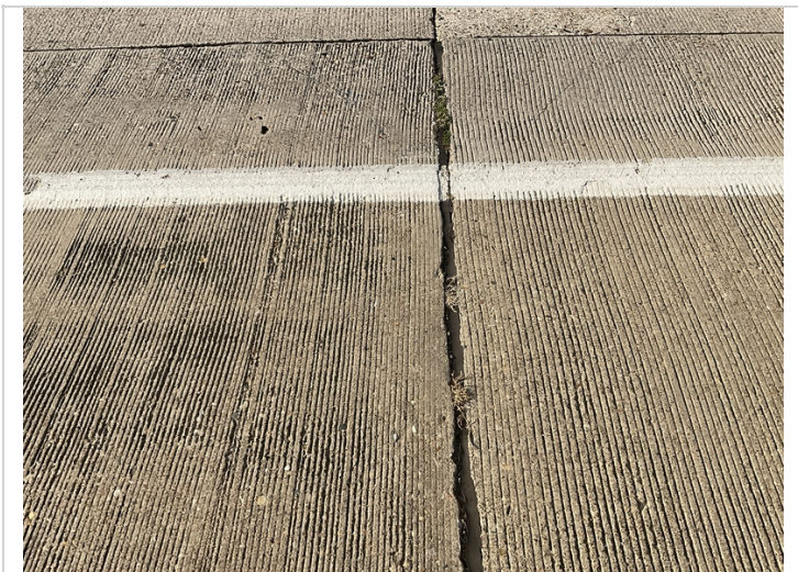
07/22 joints need cleaned and resealed
