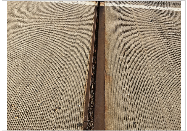
07/22 debris impacting on expansion joints
