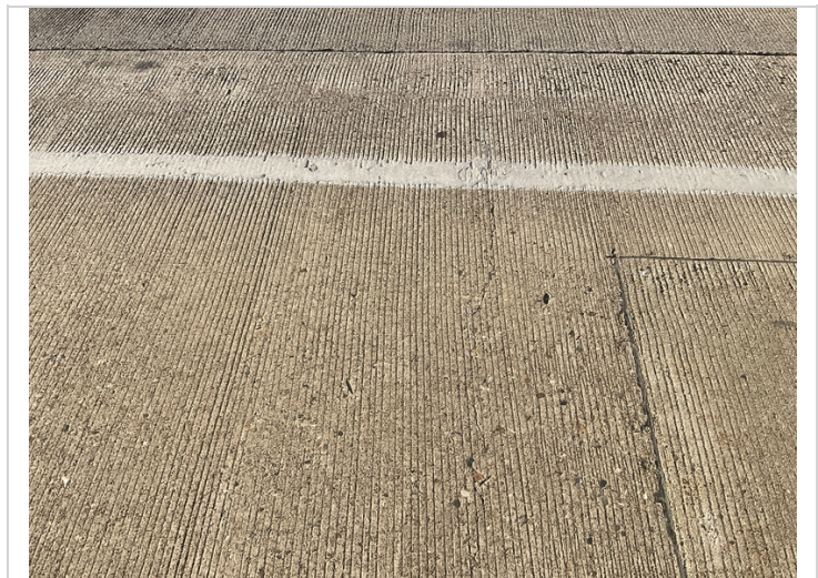
07/22 cracking in deck
